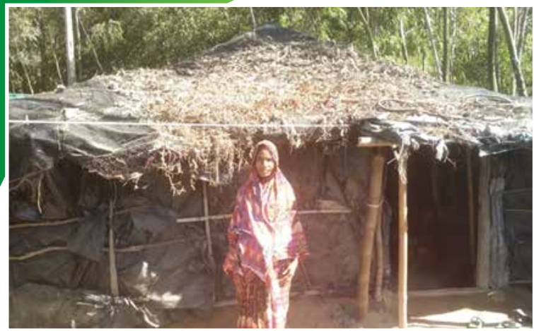
Figure 8: House made of polythene in coastal area. Photo source: Field visit, November 2022, Maheskhali, Coxsbazar.
