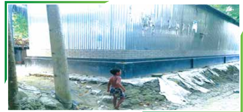
Figure 22: Local adaptation to protect houses from flood at Charrajibpur (Source: Field visit)
